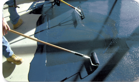
One coat application
