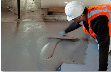
Fast setting - install most flooring in as soon as 15-20 minutes
